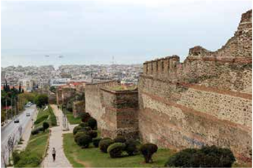
3 Thessaloniki, Part of the Eastern Walls. View from the Trigonion Tower. Source: Wikimedia Commons.
