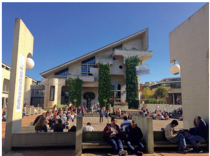
Figure 5. Iconic Place des Sciences and Science Library 1972 (arch. André Jacqmain). It was the first iconic gathering place of the University town (source: Koen Raeymakers 2018).
